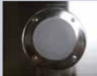
Port for CO 2 fire extinguisher
